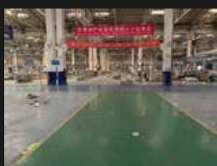
Former Linde Plant merged with Carrier
