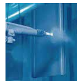
Coating treatment of external surface
